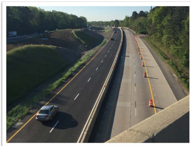
I-64 EB Traffic Shift to Phase 2 in Sections A and B
