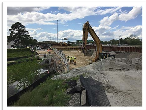
Erecting First Tiers of Wall Q
