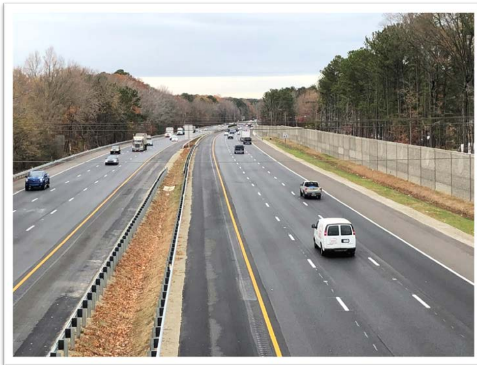
Project Site (Looking West from Denbigh Blvd.)
