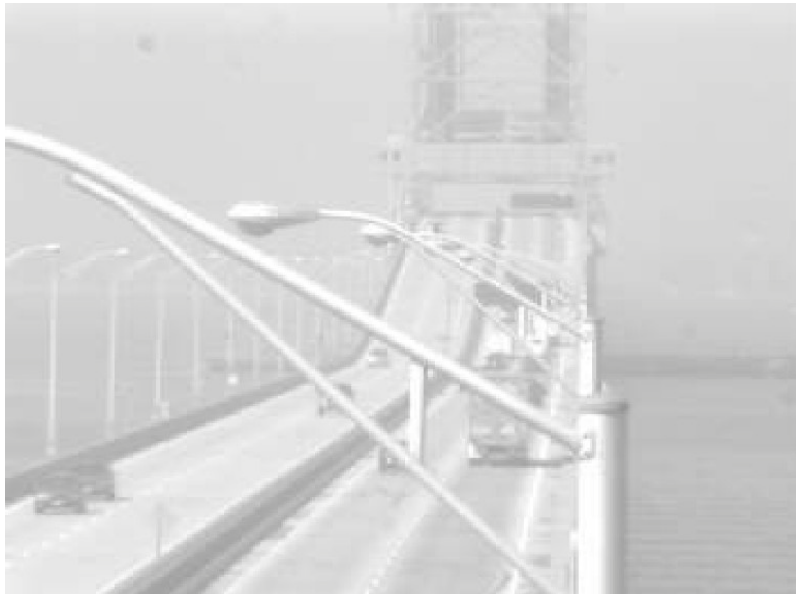
James River Bridge, 6/20/08
