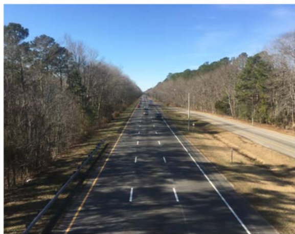
Existing facility looking westbound from weigh station
