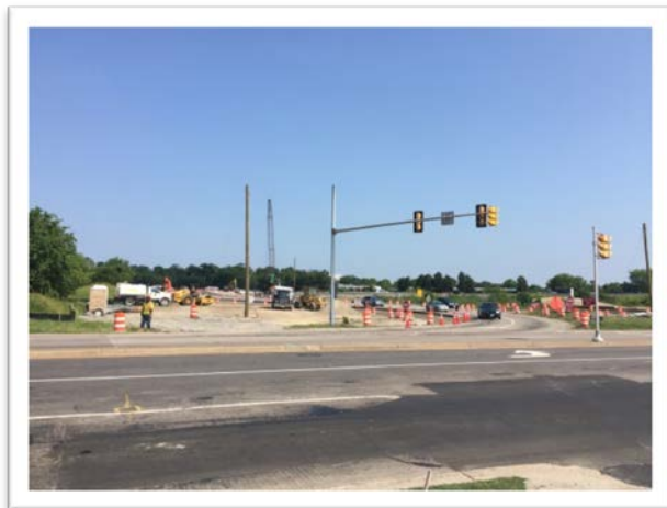
I-264 Exit 15A at Newtown Road
