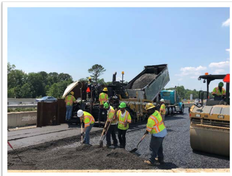
I-64 Westbound Pavement Construction at the Burma Road Bridge Approach
