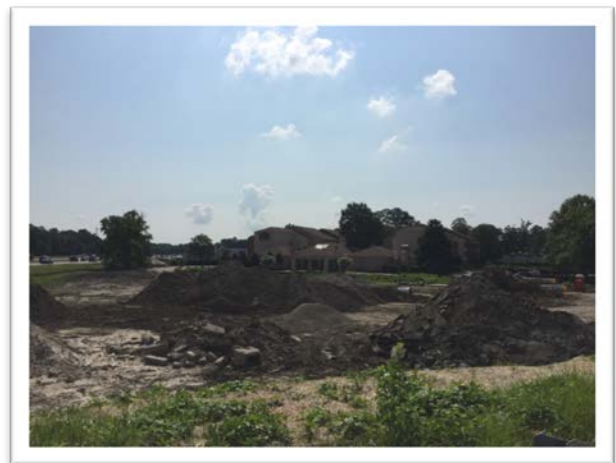
Future site of Greenwich Road Roundabout
