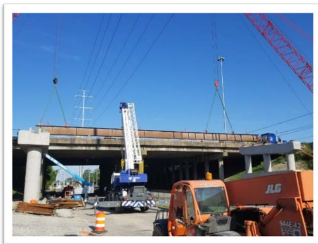
Erecting B-602 Span e Girders
