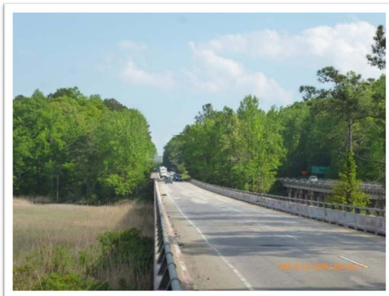
I-64 westbound looking eastbound across the Queens Creek Bridge
