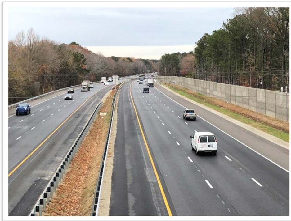
Project Site (Looking West from Denbigh Blvd.)
