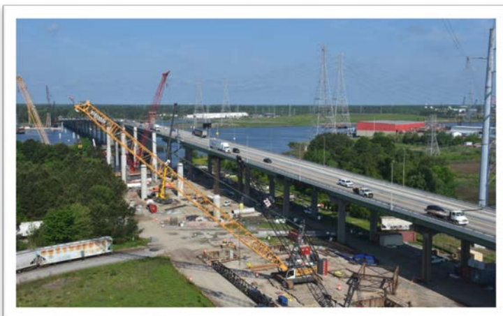
HRB Looking West
