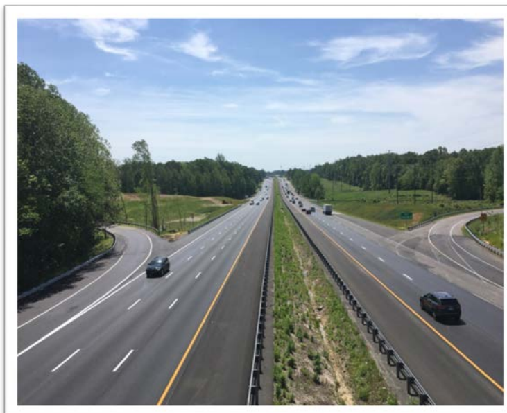
Project Site (Looking East from the Rt. 199 overpass)
