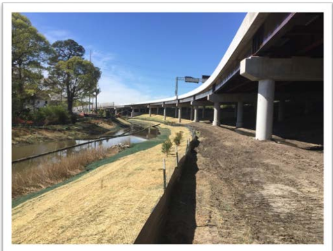
Tidal Channel Grading and Planting
