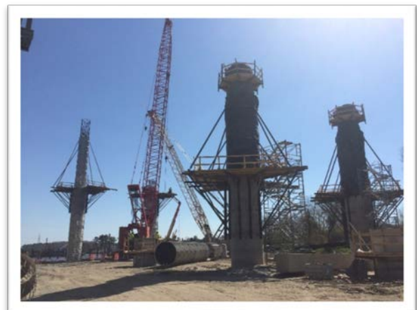
HRB Piers 20 and 21
