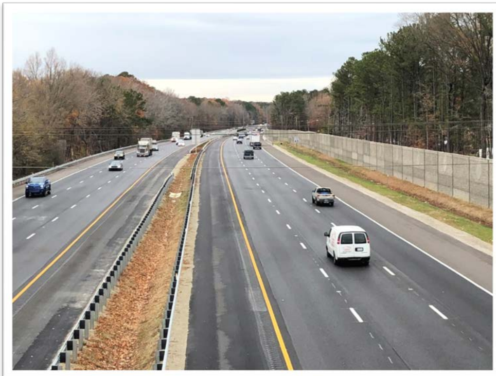
Project Site (Looking West from Denbigh Blvd.)
