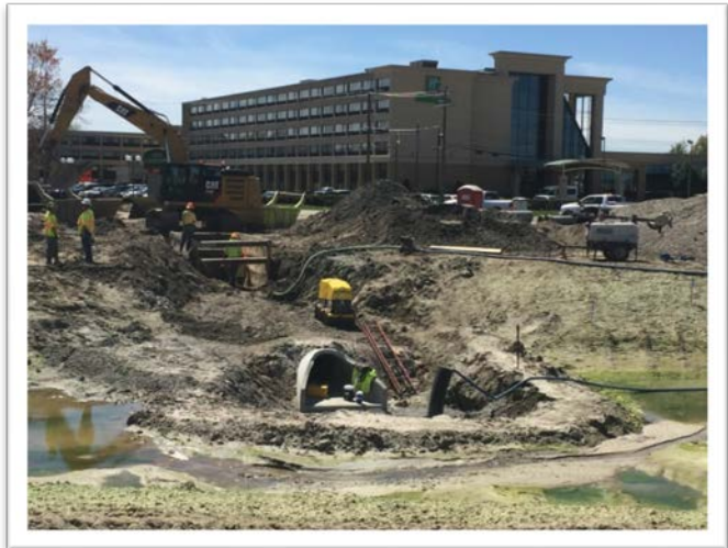
Drainage Structure Vicinity I-264 EB Exit 15B
