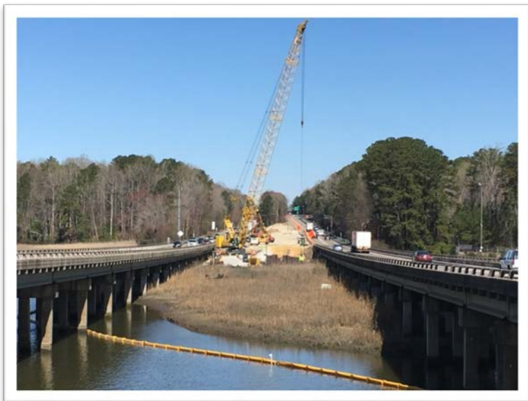
Bridge construction at west abutment of Queens Creek
