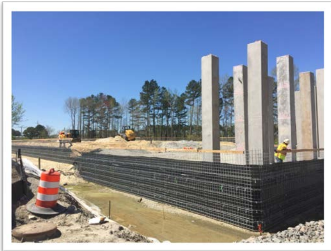
B-603; I-264 Flyover Piles Southern (Top Golf) Approach
