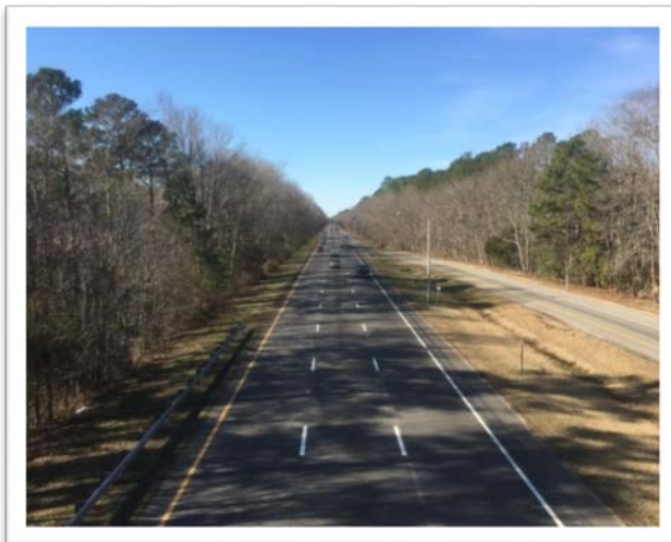
Existing facility looking westbound from weigh station
