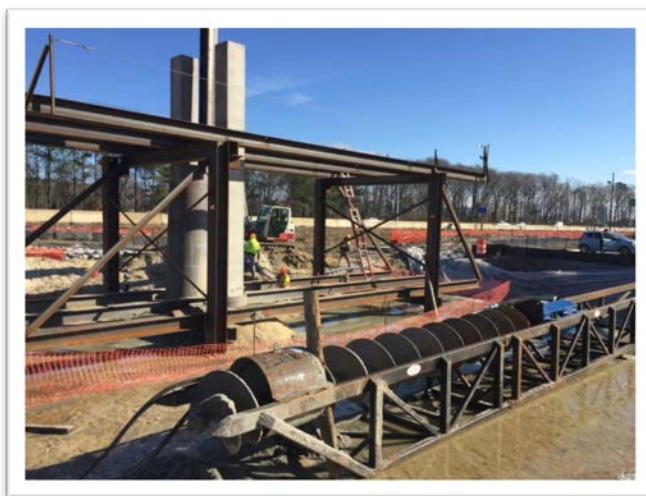
B-603 Flyover Abutment Piles (Top Golf approach)
