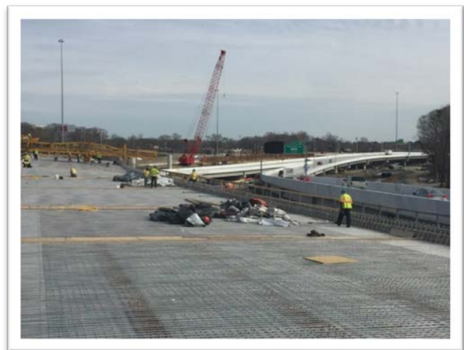
B-602 Flyover Reinforcement and Landing (background)
