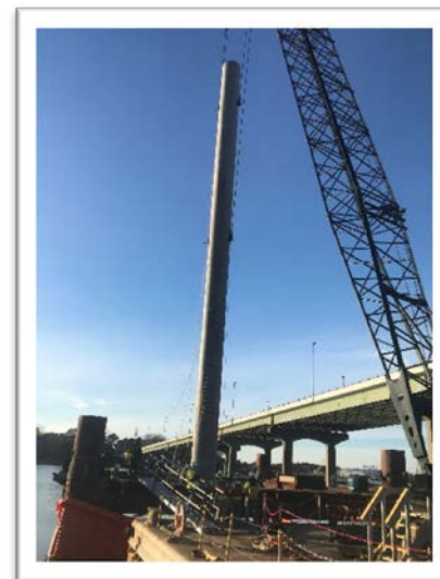
Pile Driving Operations for East Approach Spans of New High Rise Bridge
