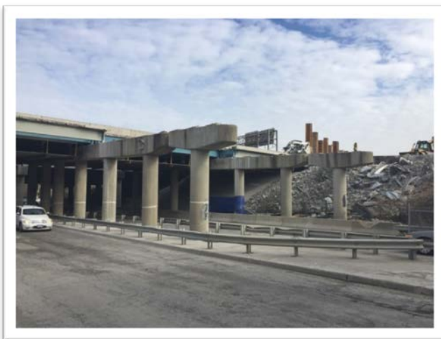
Demolition of I-264 EB over Kempsville Road
