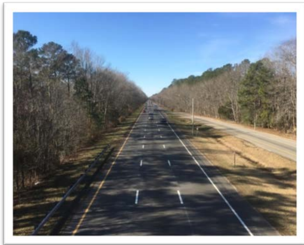
Existing facility looking westbound from weigh station
