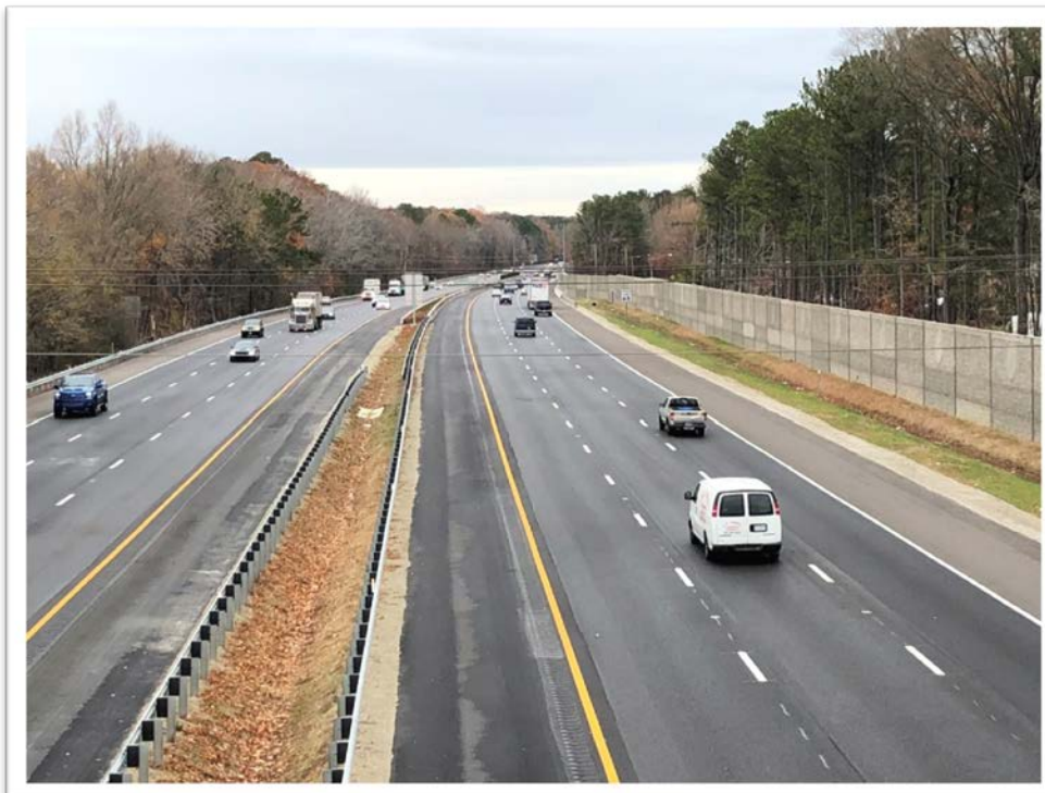
Project Site (Looking West from Denbigh Blvd.)
