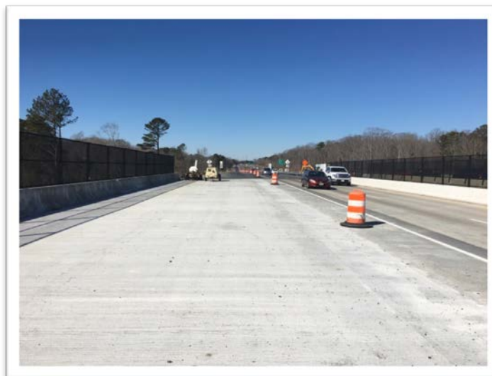
Eastbound I-64 latex concrete overlay at the Burma Road bridge
