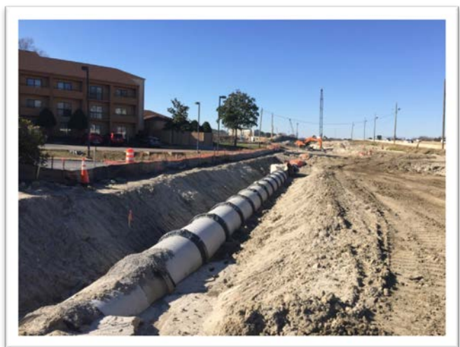
Installed drainage pipe parallel to Courtyard Marriot
