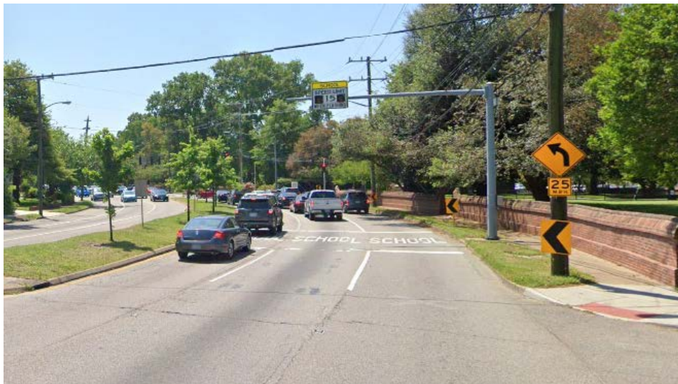
FIGURE 94 Existing Chevron Alignment Signs on the Southbound Lanes of Hampton Boulevard between Brunswick Avenue and Bolling Avenue
