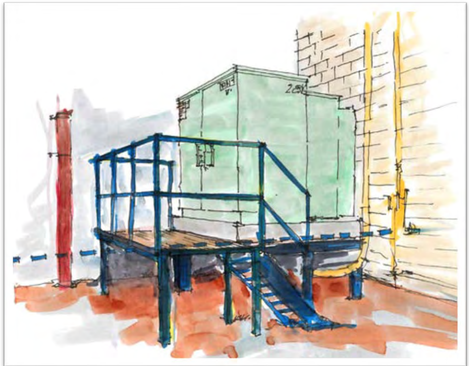
Figure 4. Elevated electrical substation. Source: Resilient Industry Mitigation and Preparedness in the City's Industrial Floodplain .
