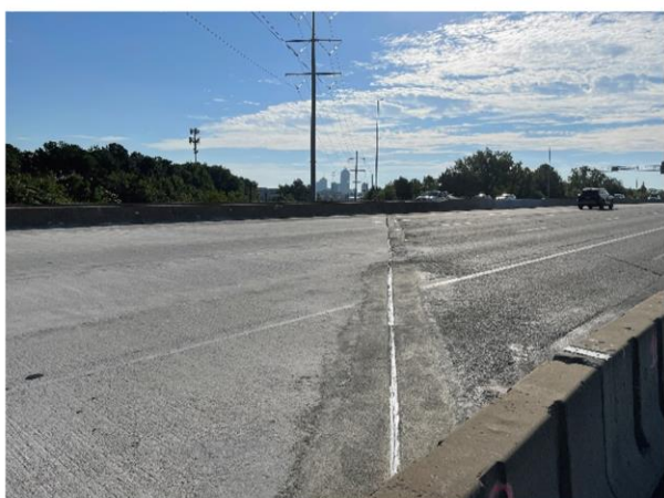
Existing B602 Expansion Joint Reconstruction in Progress
