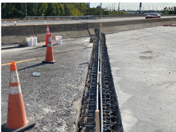
Final Section of Expansion Joint Reconstruction
