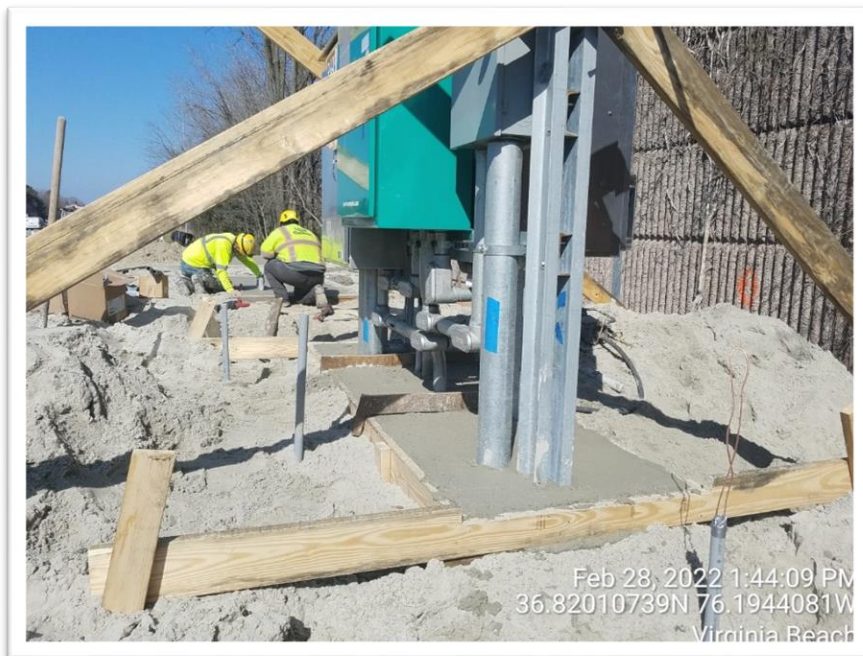
Equipment Pad at Backup Generator Site 64-105
