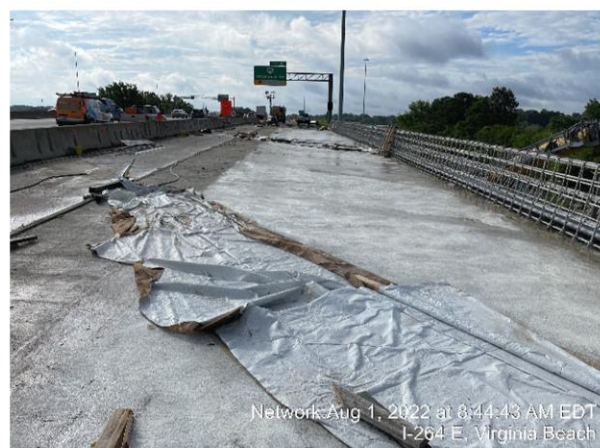
B602 Widening – Deck Placed, Closures Curing
