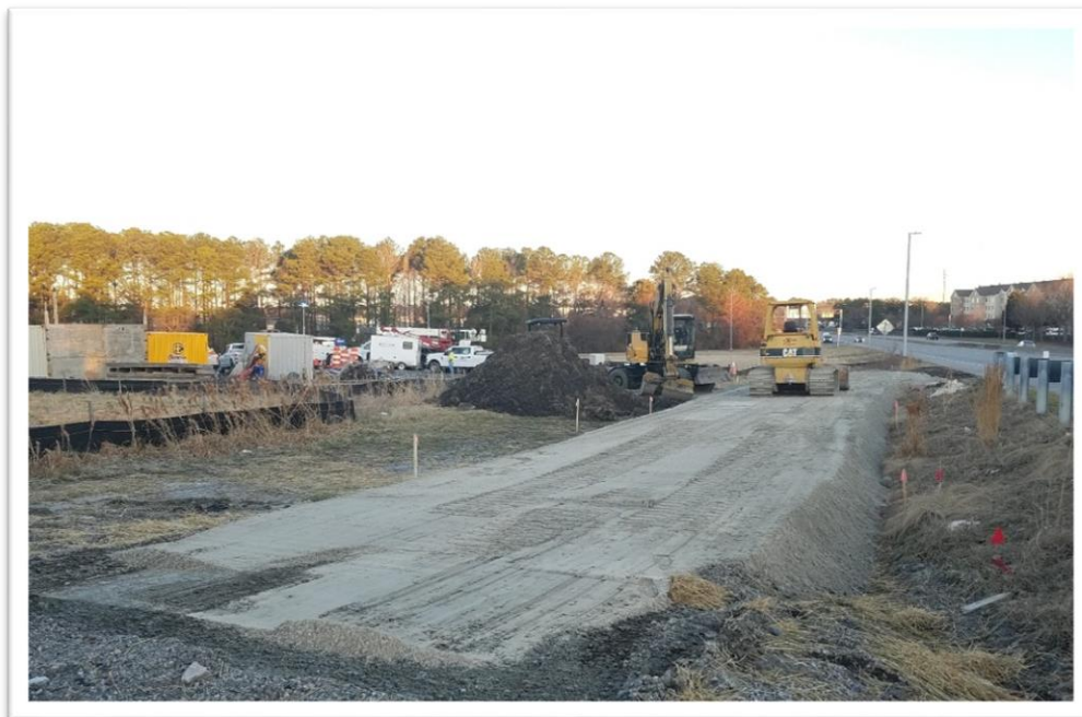
Equipment Pad at Backup Generator Site 64-104
