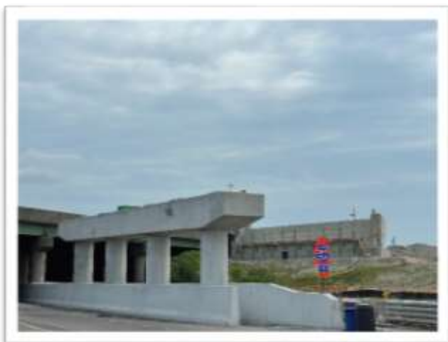
Newtown Road Bridge Center Pier and East Abutment
