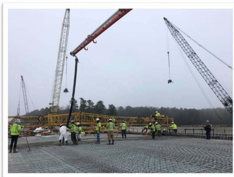
Concrete bridge deck placement at the EB Queens Creek Bridge
