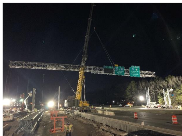
Overhead Sign Structure east of Top Golf Installed
