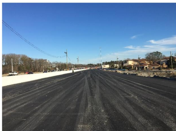
Base Mix Asphalt Complete on CD Lanes East of Newtown
