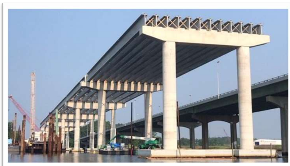
Girder Erection Completed on Spans 6 to 10 (Looking West)
