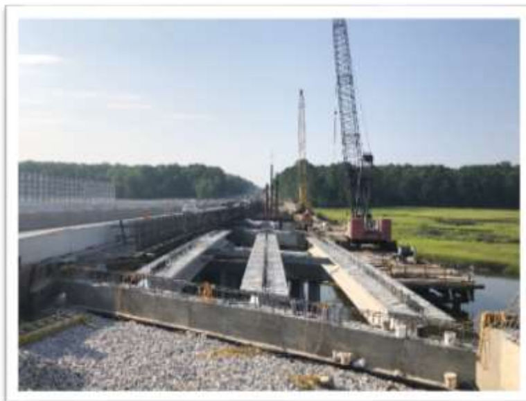
Concrete beam installation at the Westbound Queens Creek Bridge
