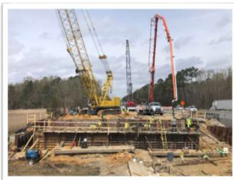
Eastbound Queens Creek Bridge Abutment Construction
