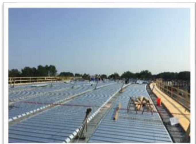
Stay in Place Forms and Overhangs on Flyover Bridge
