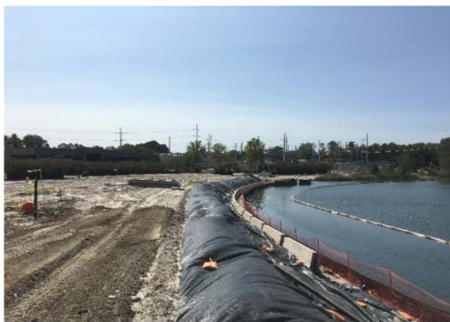
Surcharge Complete at B621 Approach to Flyover
