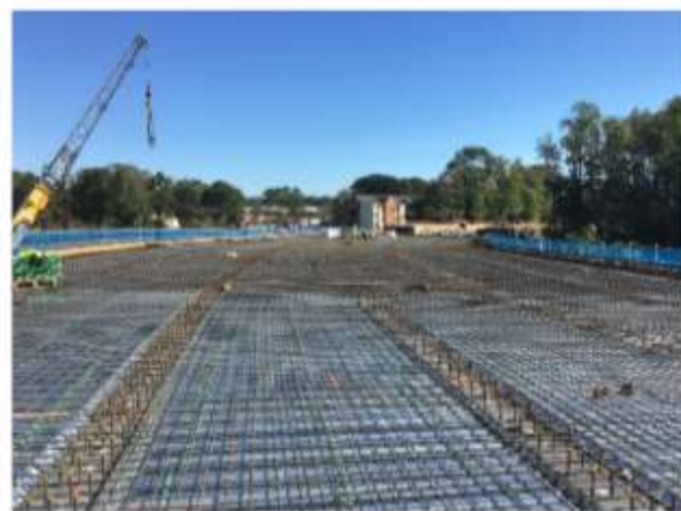
Deck Reinforcing Steel on Flyover Bridge
