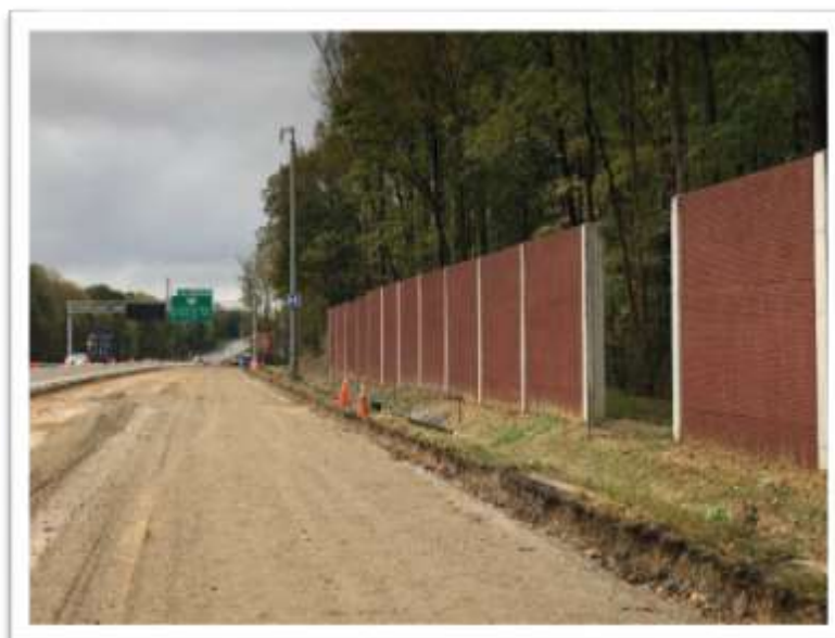
Eastbound noisewall construction on east end of project
