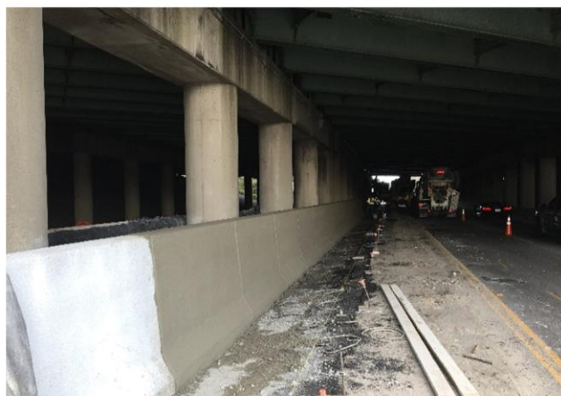
Newtown Bridge (B601) Bridge Pier Protection Barrier
