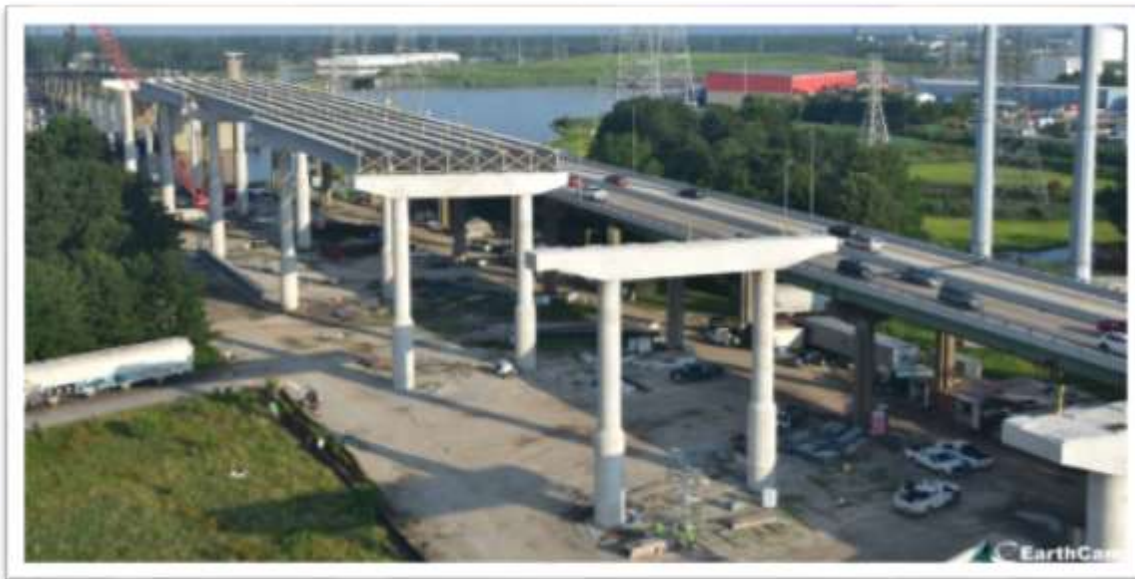
HRB – Piers 19-25 (Looking West)
