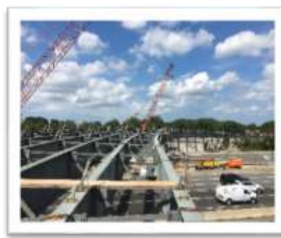
Greenwich Road Flyover Steel Spanning I-264
