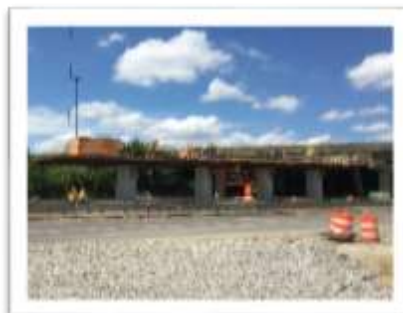
Bridge Widening over Newtown Road
