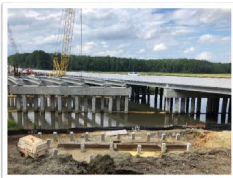
East Abutment of the new EB I-64 bridge over Queens Creek
