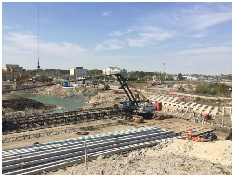
West end of project limits Newtown and Greenwich Roads Intersection Showing Storm Water Management Pond and Ground Improvement Piles
