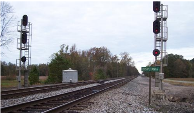
Photo 2: New Bi-directional signaling system at Disputanta, VA.
