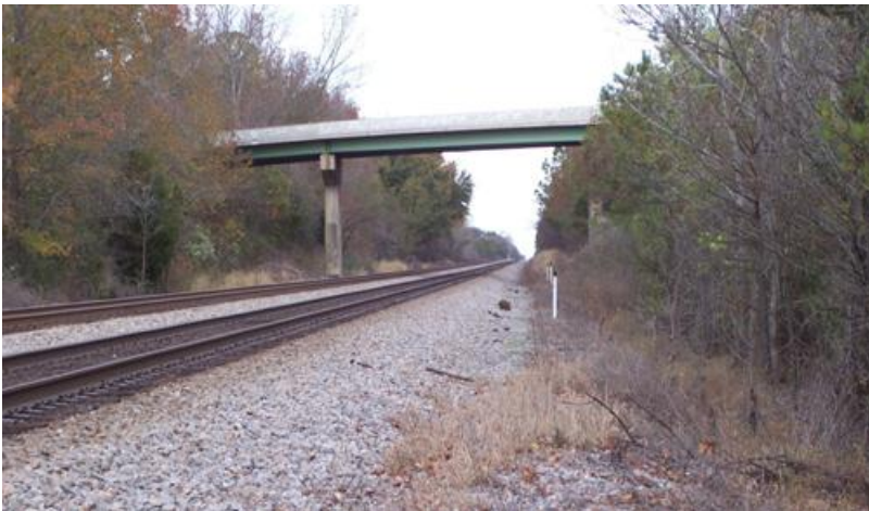
Photo 9: Bridge at Disputanta, VA allows room for one track at 14 feet center, but not two tracks or wider separation. This bridge may have to be replaced to allow room for additional tracks.
