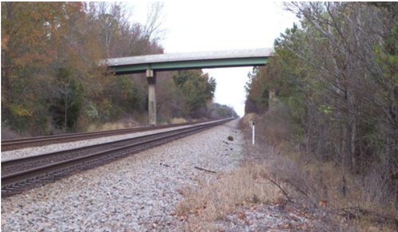
Photo 9: Bridge at Disputanta, VA allows room for one track at 14 feet center, but not two tracks or wider separation. This bridge may have to be replaced.
