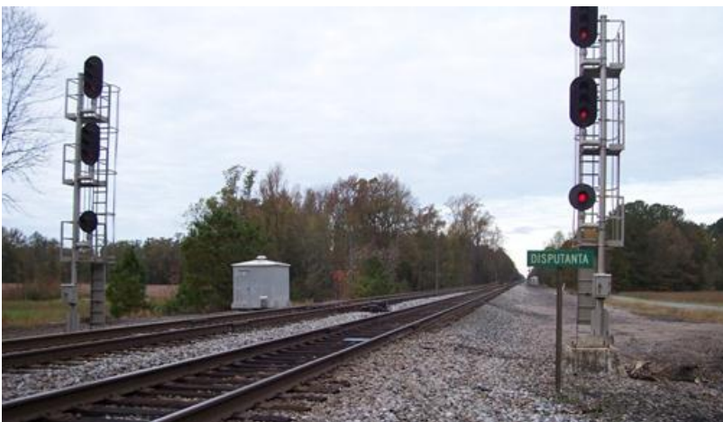
Photo 2: New Bi-directional signaling system at Disputanta, VA.
