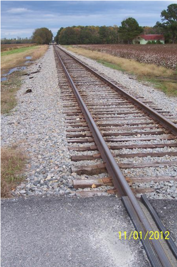
Photo 28: Welded rail on NS line from Franklin to Suffolk.
