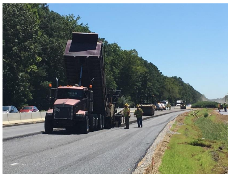
Asphalt and CCPRM placement westbound I-64 median
