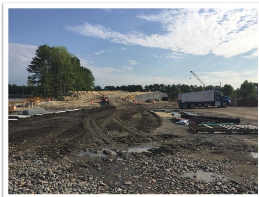
Constructing MSE Wall; Top Golf approach to I-264 Flyover
