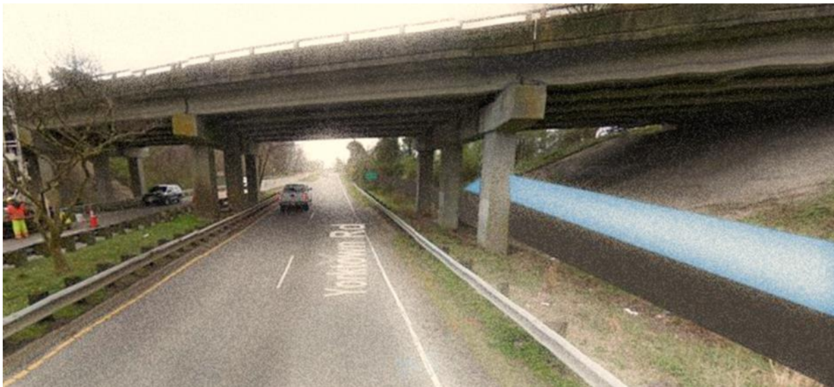
The existing retaining walls in the I-64 underpasses (like the Yorktown Road example above) would need to be reconfigured to accommodate a 10' shared-use path. The blue area above approximates the area of the retaining wall that would require modification.
