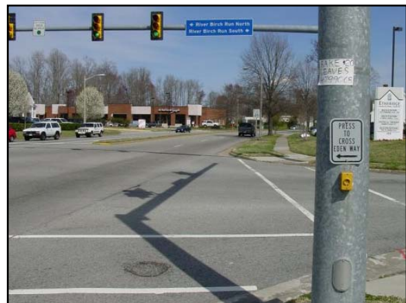
Pedestrian push buttons and crosswalks currently exist for two approaches of the intersection of Eden Way and River Birch Run; however, no pedestrian signals are present to alert pedestrians when it's safe to cross.
