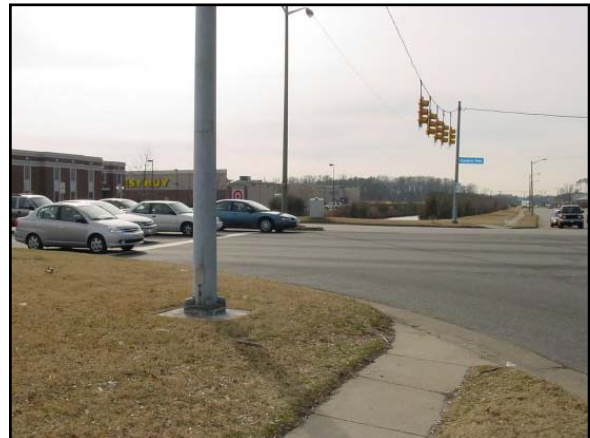
Looking west across Greenbrier Parkway at Eden Way. Sidewalks lead to the intersection on both sides of Eden Way, but no crosswalk or pedestrian signal is provided.
