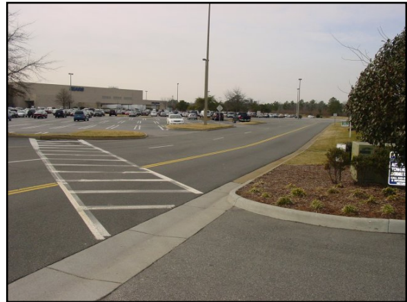
Mall Ring Road location connecting senior residential area to the northeast parking lot at the mall. Needs curb ramp for persons in wheelchairs and sidewalks leading up to the existing crosswalk.
