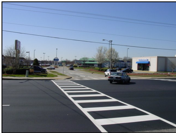
An example of a high-visibility (ladder bar marking) crosswalk used in Virginia Beach.
