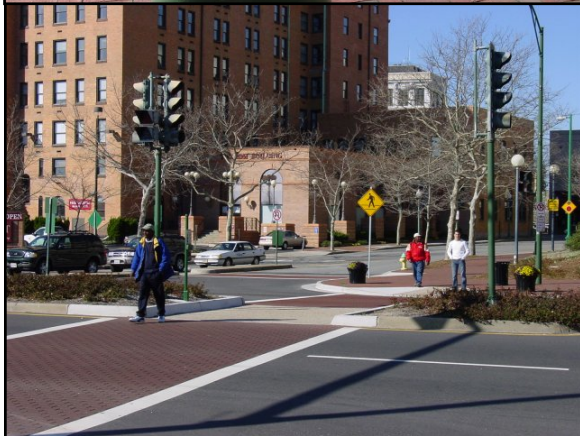
An excellent example of a mid-block crosswalk treatment (located across Waterside Drive in Downtown Norfolk). Features include a high-visibility crosswalk, clear instructions on push button locations, and pedestrian signs and signals.
