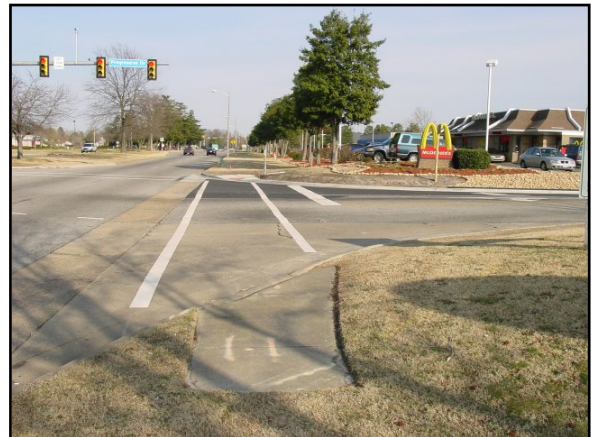
Incomplete sidewalks at the intersection of Volvo Parkway and Progressive Drive
