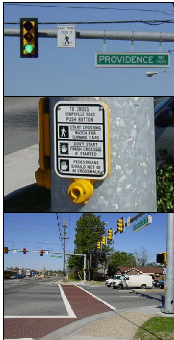
The intersection of Kempson Road and Providence Road in Virginia Beach contains many characteristics recommended for the Greenbrier Parkway and Crossways Boulevard/Mall Main Entrance intersection, such as stamped asphalt crosswalks, pedestrian signals, and overhead signs.
