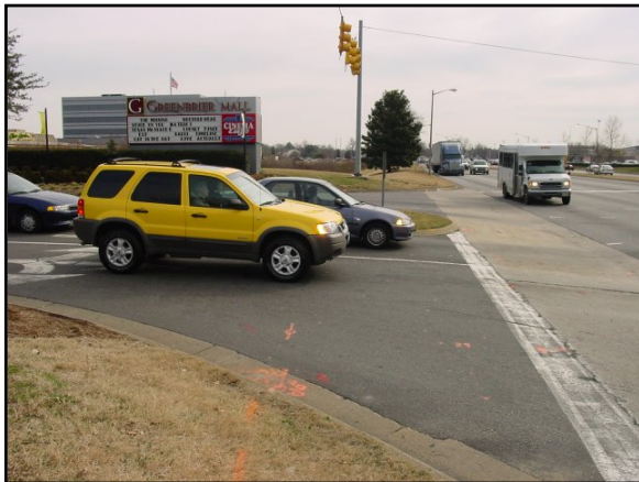
Greenbrier Mall driveway entrances do not have crosswalks or median refuges for pedestrians to safely cross.
