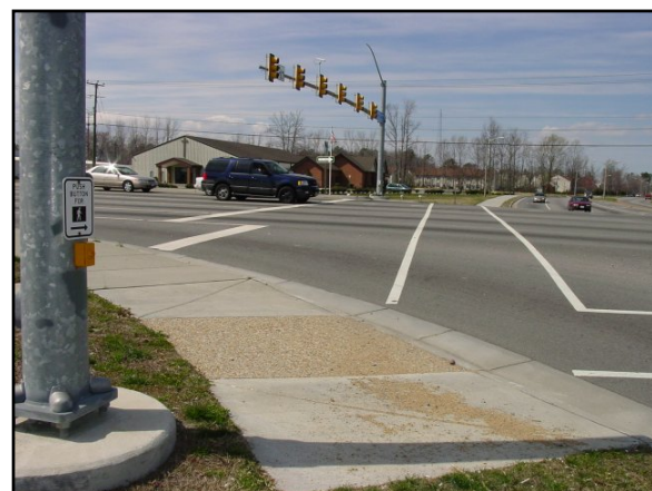
Horizontal bar crosswalks with pedestrian push buttons are currently used at the intersection of Greenbrier Parkway/Butts Station Road and Kempsville Road in Chesapeake. No pedestrian signals are used, however.
