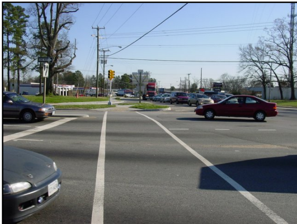
Horizontal bar crosswalks and pedestrian signals with push buttons are currently used at the intersection of Kempsville Road and Battlefield Boulevard in Chesapeake.
