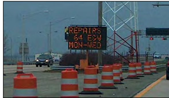
PICTURE 7 – Temporary Variable Message Signs could be used on northbound I-564 to alert commuters of the delay at Gates 3/3A.
