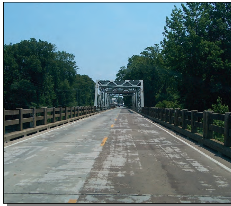
PICTURE 4 – The Route 35 bridge over the Nottoway River in Courtland is classified as functionally obsolete. Functionally obsolete bridges are those bridges that don't meet current design standards.
