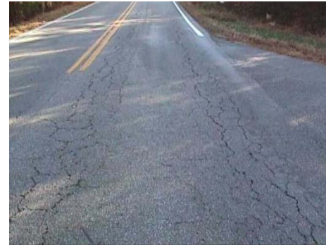
Figure 5 Cracking
