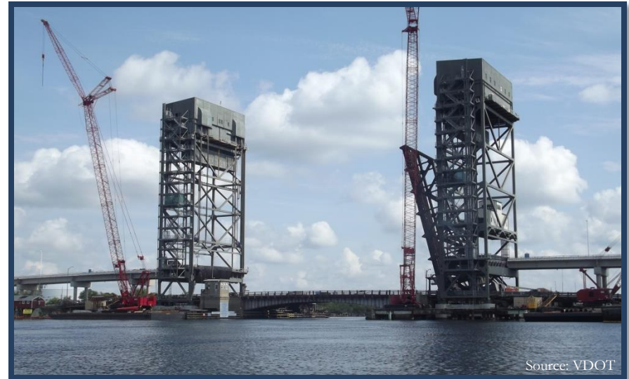
Construction of the Gilmerton Bridge in Chesapeake, VA
