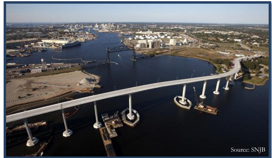
South Norfolk Jordan Bridge in Chesapeake, VA
