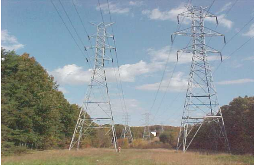
Photo 3 - Dual Lattice Tower Configuration
