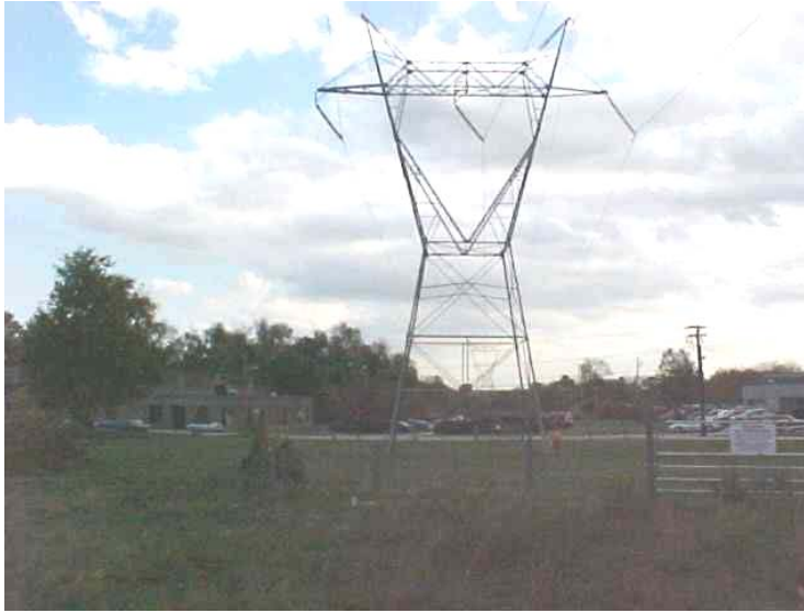
Photo 5 – ‘Short and Wide’ Lattice Tower
