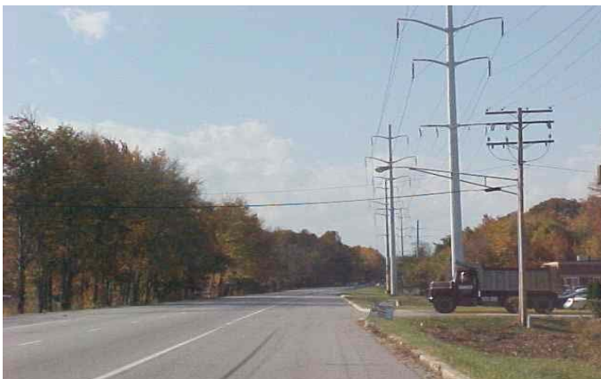
Photo 2 - Steel Pole in Tangent Section
