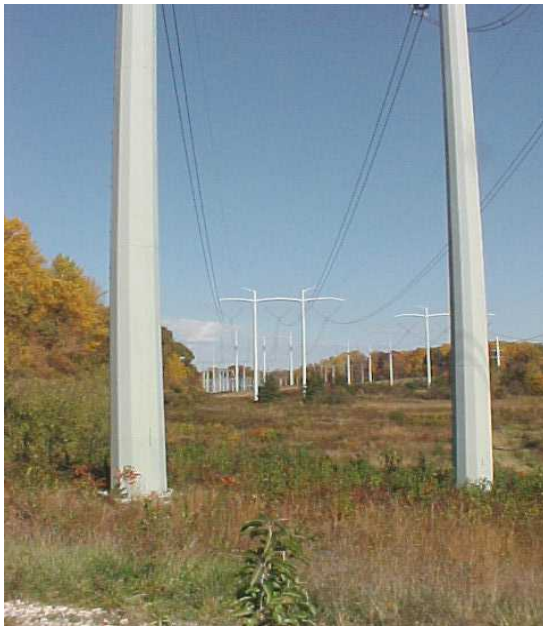
Photo 6 - Steel Poles Supporting 500kv Wires
