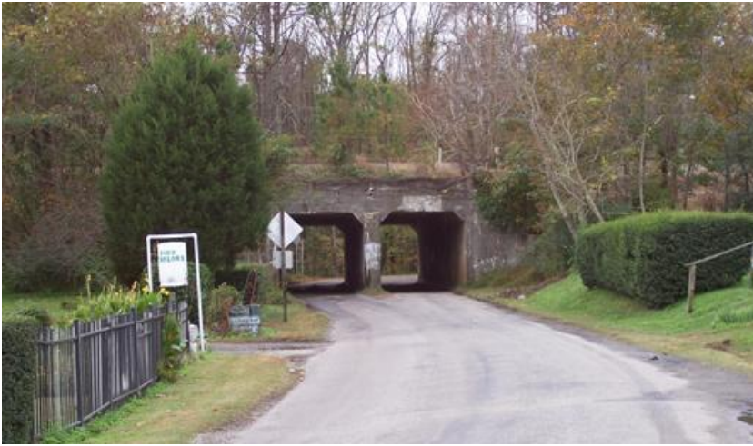
Photo 5: Overhead rail bridge on Golf Course Drive at Disputanta, VA would have to be widened or replaced.
