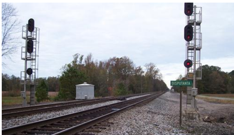
Photo 2: New Bi-directional signaling system at Disputanta, VA.
