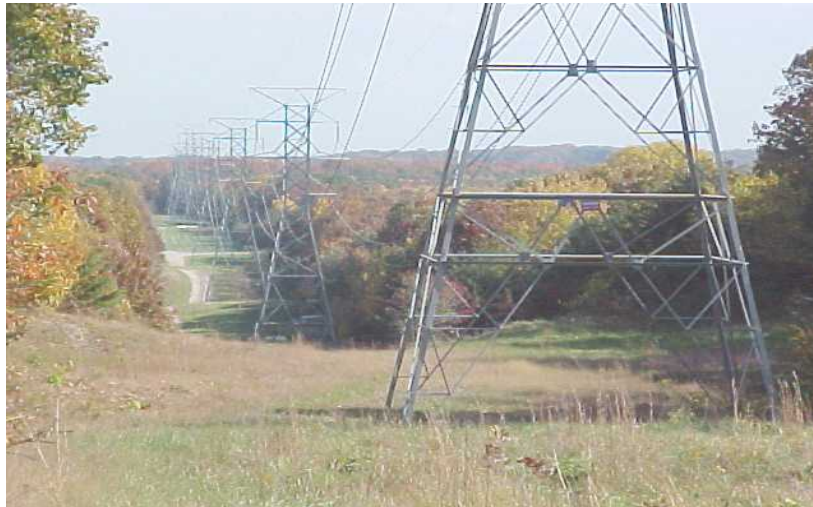
Photo 4 - Single Lattice Tower Configuration
