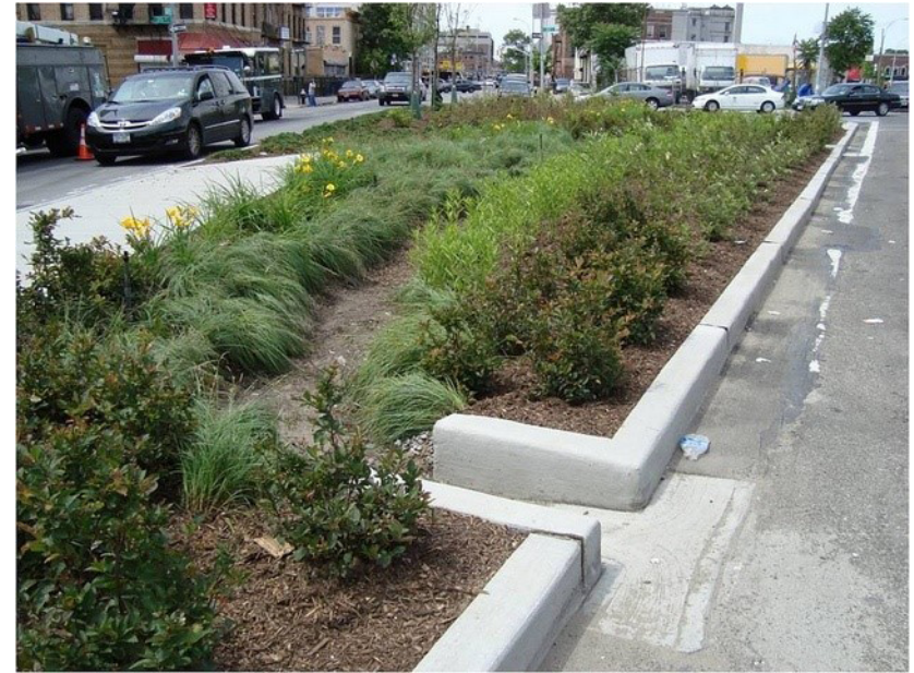
Roadside Bioretention Practice
