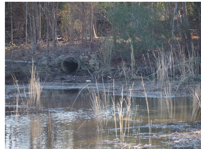
Stormwater Outfall
