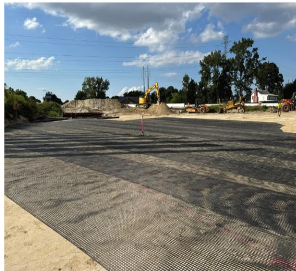
Geogrid and Fill Placement at B679
