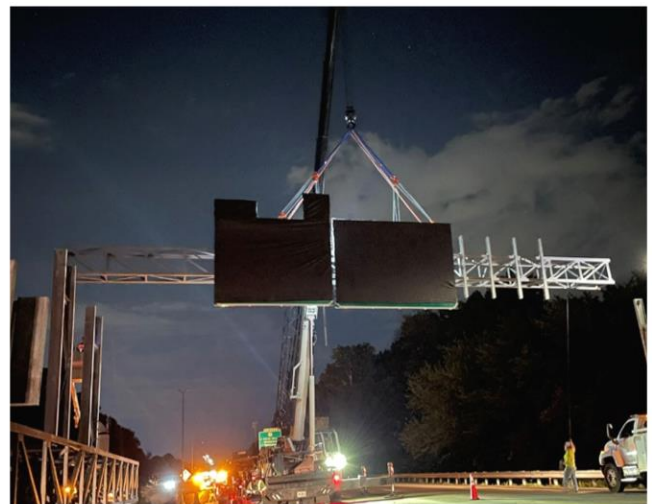
Overhead Sign Structure Installation
