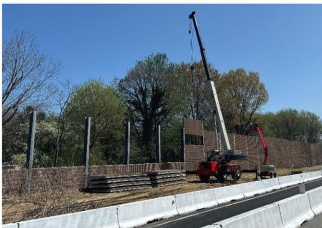
Ramp A Noise Wall Demolition
