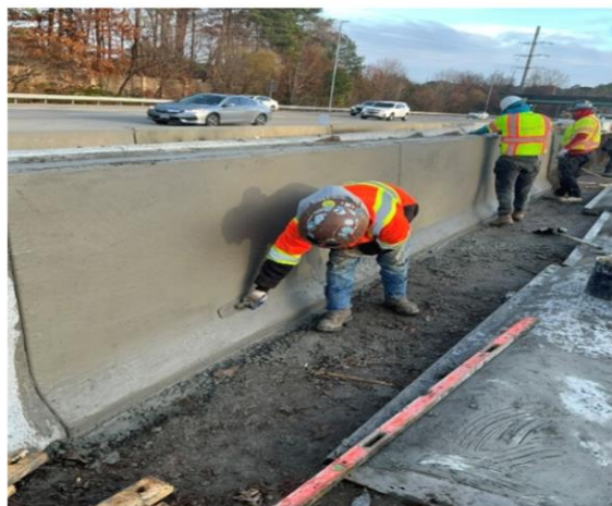
I-64 Median Barrier Placement
