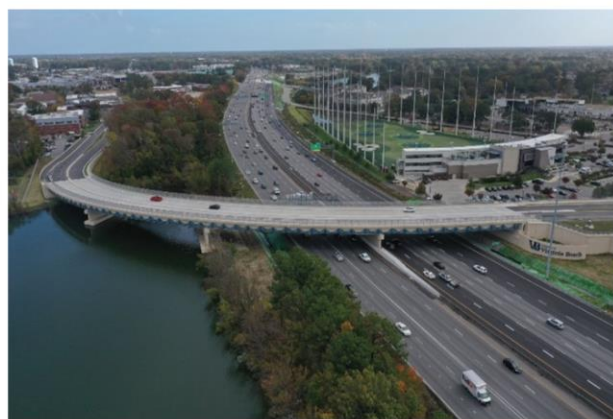
I-264 EB at Cleveland Street Flyover
