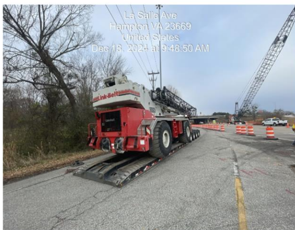
Two New Cranes Delivered for Bridge Construction
