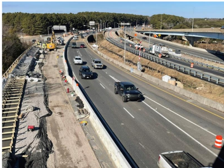
Widening along I-64 EB near I-564 and work in the Reversible Lanes
