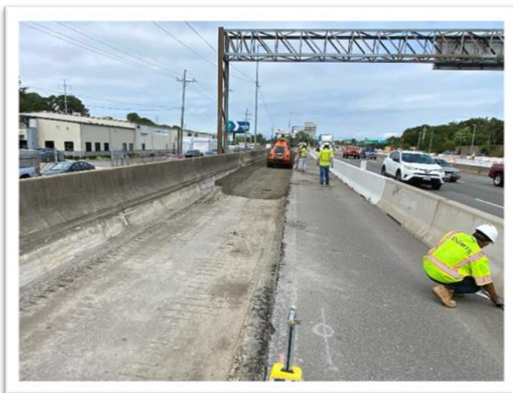
Cement Treated Aggregate placement along median barrier
