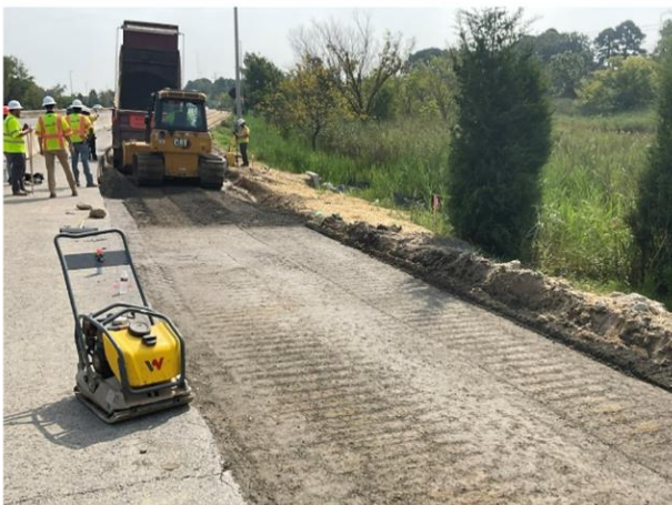
Placement of Cement Treated Aggregate I-64EB
