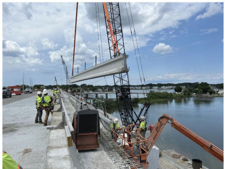
HREL 4C setting of beams on the WB I-64 bridge over the Hampton River
