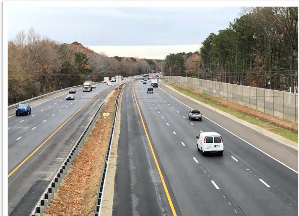
Project Site (Looking West from Denbigh)
