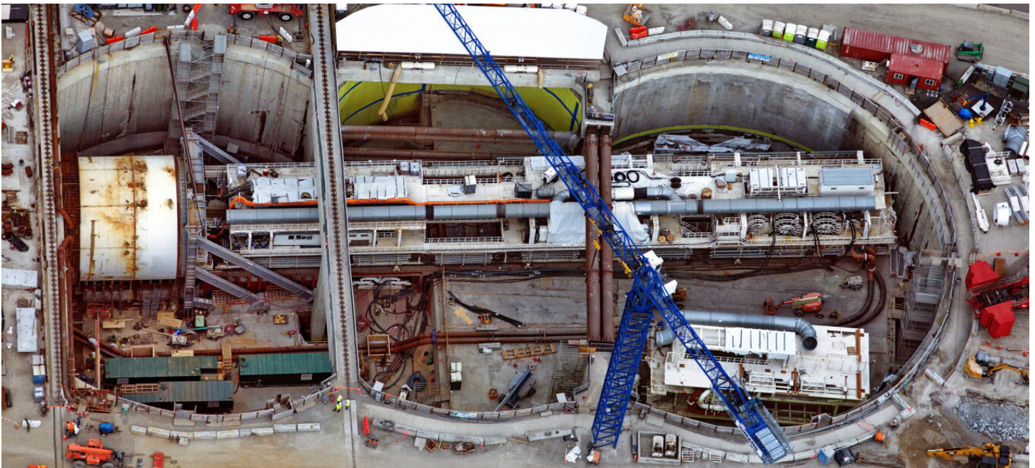
Figure 2. Tunnel Boring Machine for the Hampton Roads Bridge Tunnel
