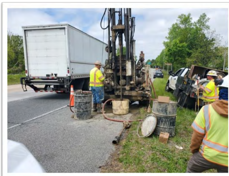
Supplemental Borings on Exit 291 Ramp
