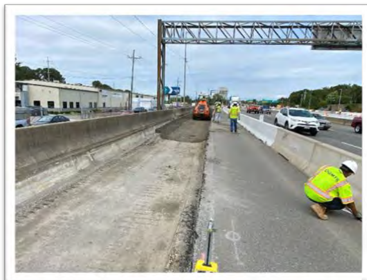
Cement Treated Aggregate placement along median barrier
