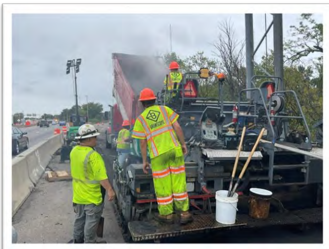
Asphalt Placement I-64 EB Outside Shoulder
