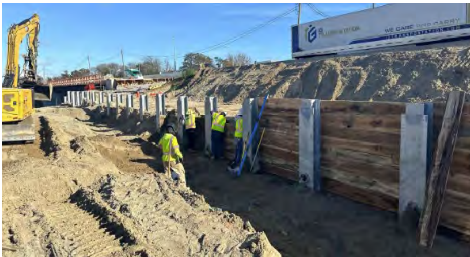
◀ Retaining Wall 310 near 4 th View St. Auger cast piles and lagging.
